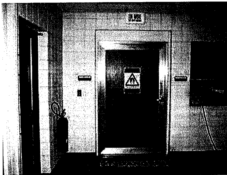
(4) This door is a typical style door that leads into the magnet room. For most MRI scanners, the 5-G line is inside the door, so tools and equipment can be safely brought just to the area outside the door.
