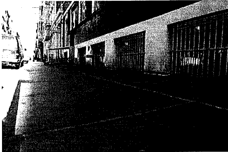
(14) Synthetic windows along the base of a South of Houston Street (SOHO, NYC) building provide natural light to below-grade areas.
