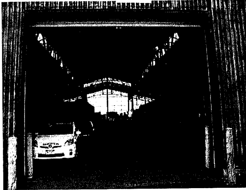
(8) An inside view of the New York City Sanitation garage, which has a lightweight steel truss-supported roof monitor.
