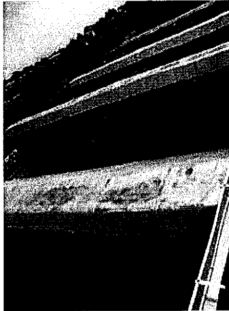
(6) Vertical glazing, sloped roofing material, and valley gutters are major components of a sawtooth roof.
